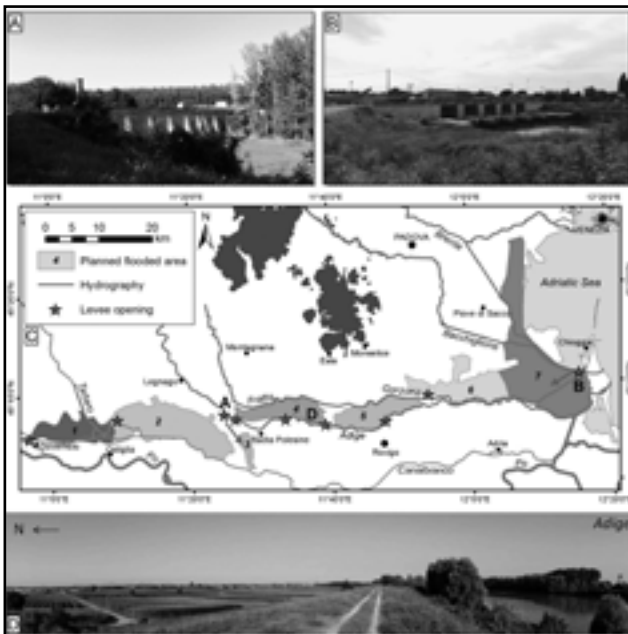
Figure 6. Examples of hydraulic structures that would be used to manage the 1918 planned flood in the Southern Venetian Plain A) Rosta Castagnaro spillway; B) Bacchiglione water gate near Chioggia; C) map showing the planned flooded areas and the levee openings along rivers and canals. The two arrows show the direction of the waters from the two water gates in A) and B); D) landscape view of the fields north of the Adige River (on the right): note the supraelevated river “over” the lands.
