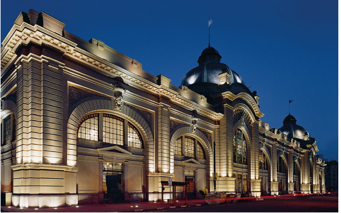
38. The main façade of the Central Market of São Paulo City at night, photo by Andrés Otero.
