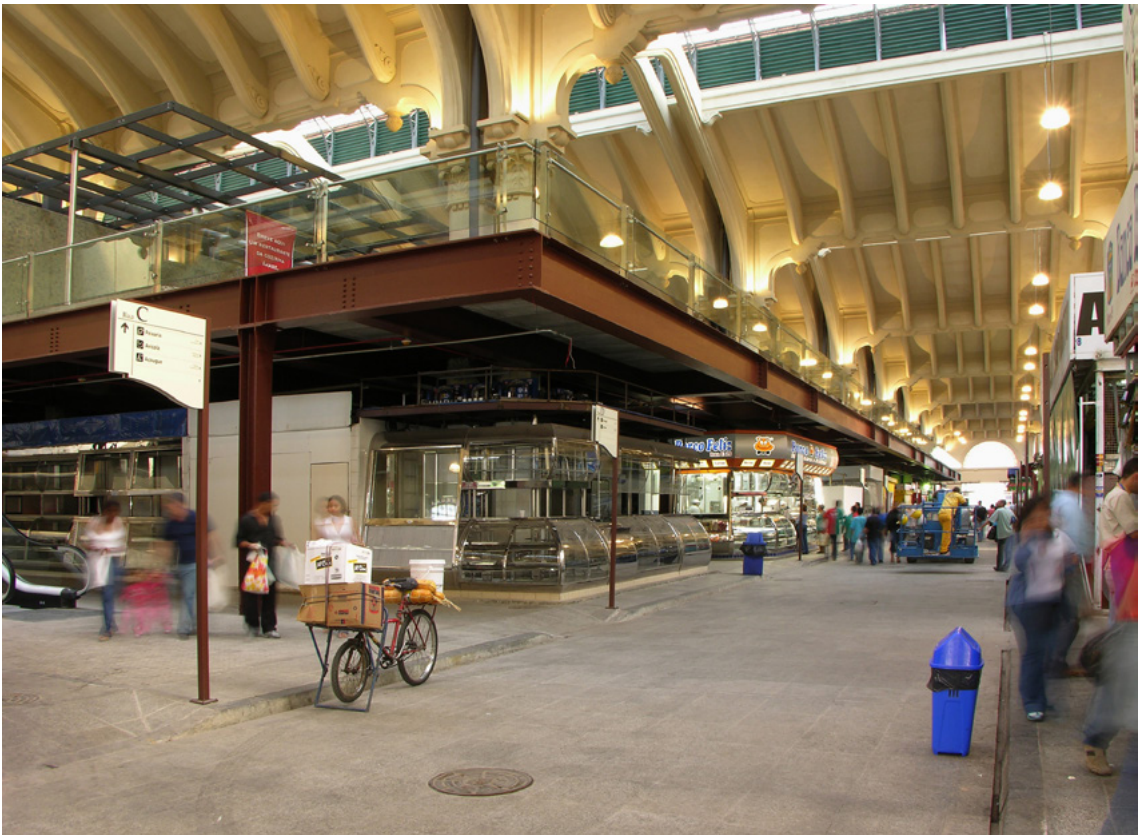
41. The mezzanine introduced inside the market, photo by Marcelo Scandaroli.
