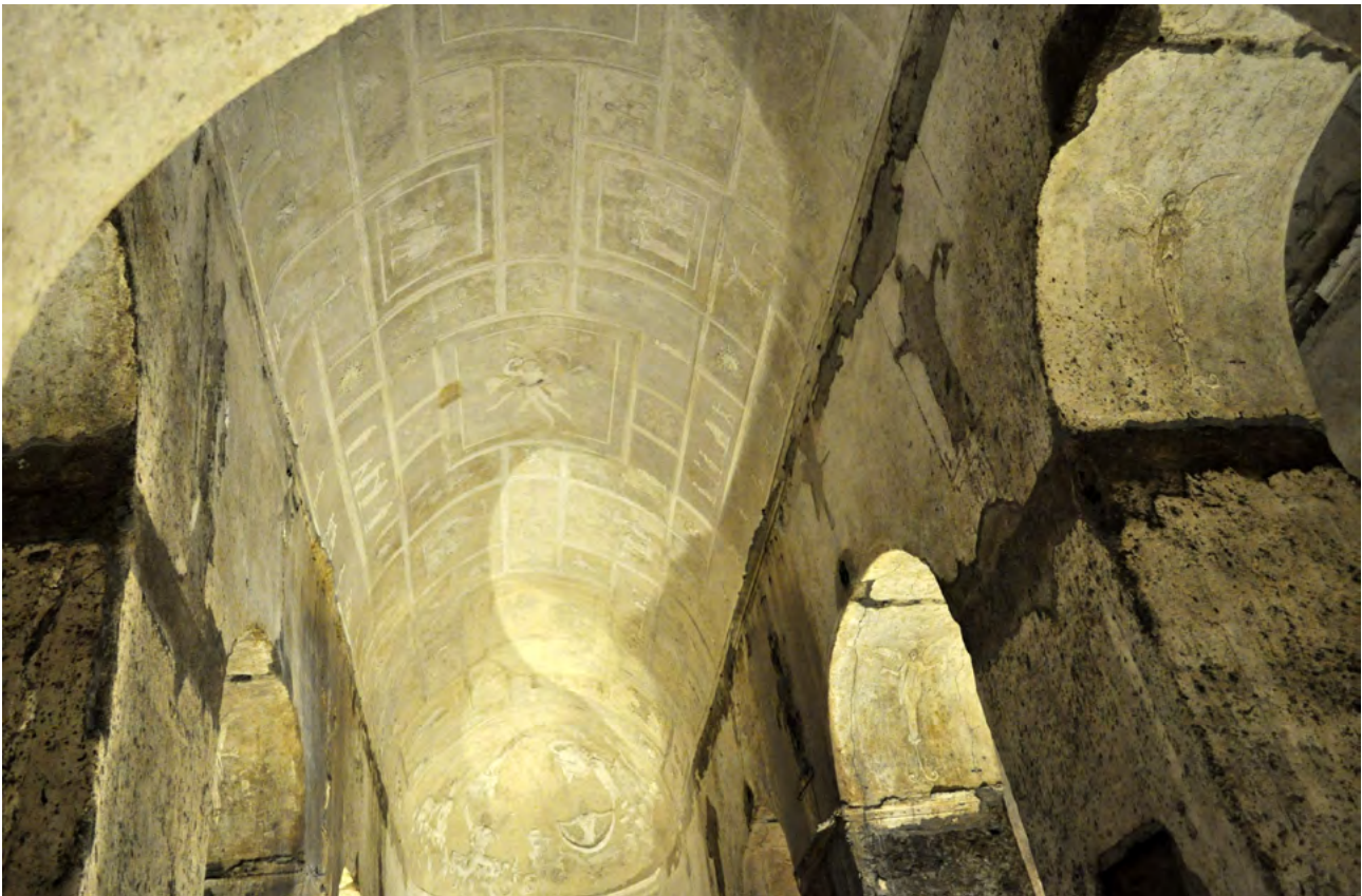
The tunnel vault of the central nave with a scene 'the rape of Ganymede' in the central square.
