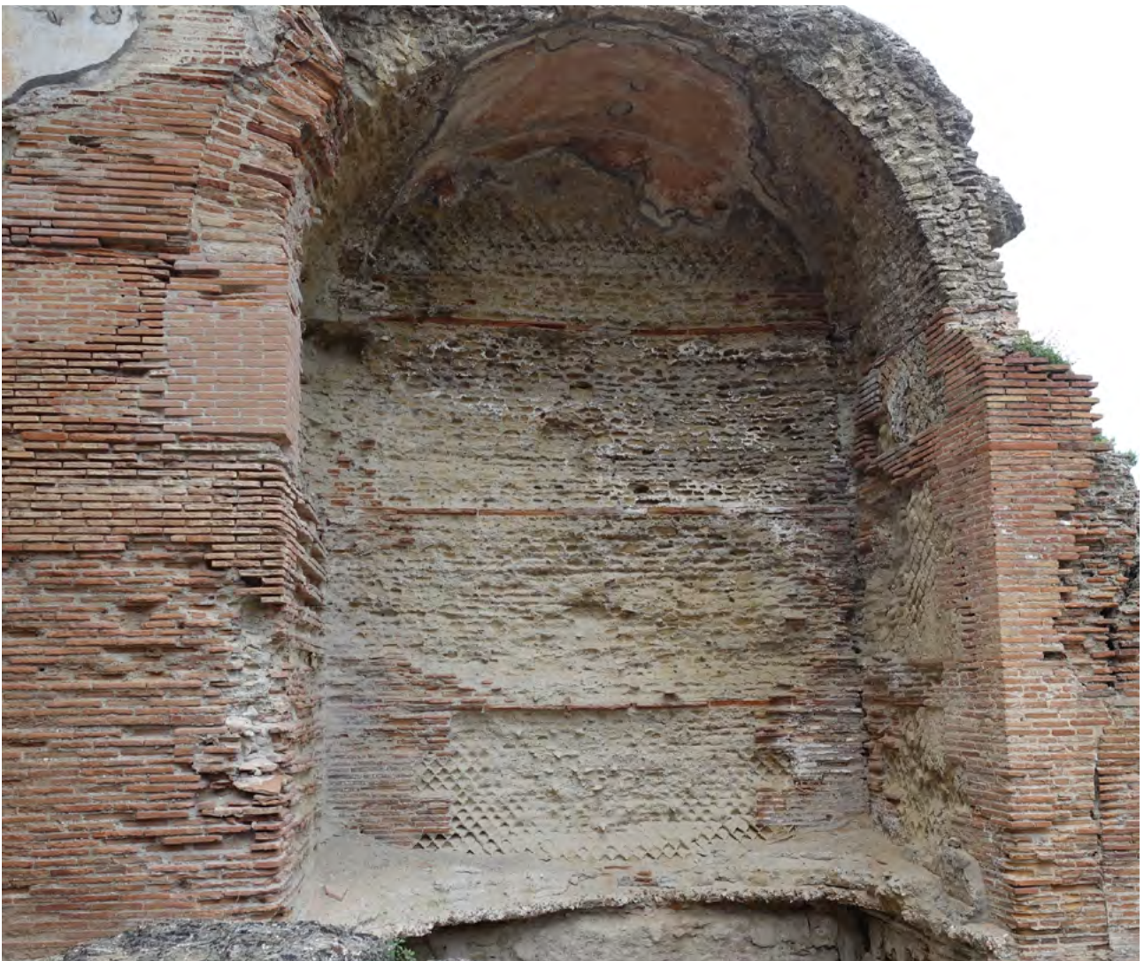
Baiae , sector L, room 33 with remain of wall painting.
